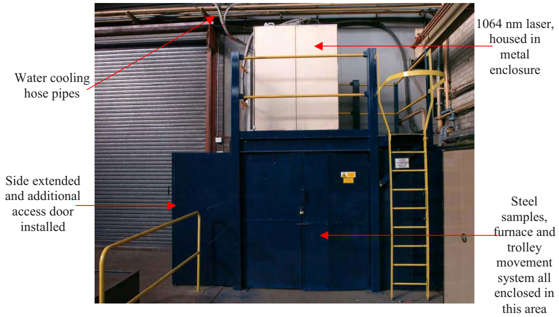
Fig. A1.1: Extended laser containment area at Corus Teesside Technology Centre (2006)
