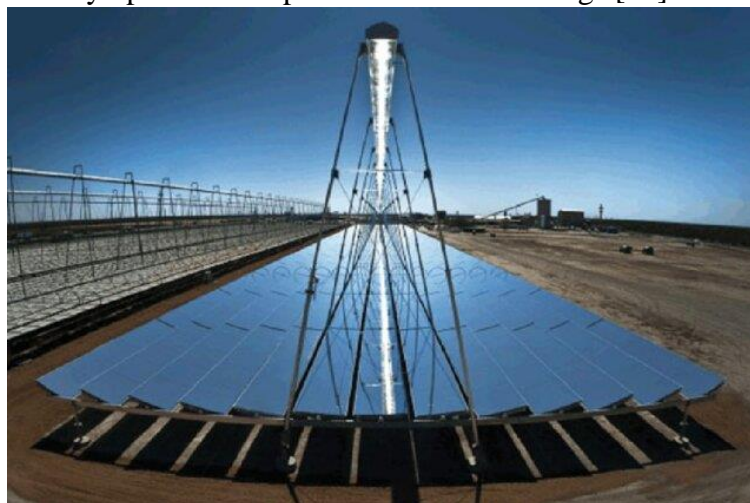
Figure 2.9 Linear Fresnel reflector (LFR) [29] (with permission from copyright owner)
