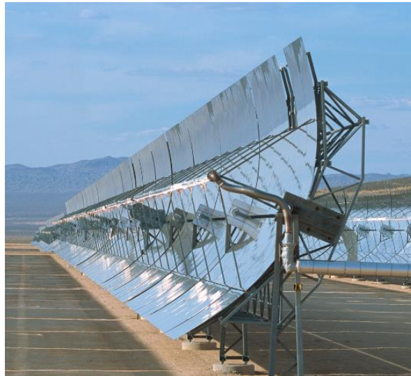
Figure 2.14 Parabolic trough collectors
