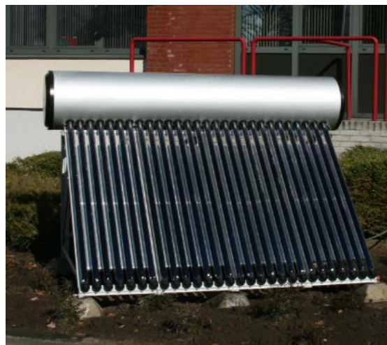
Figure 2.7 Evacuated tube solar collector
