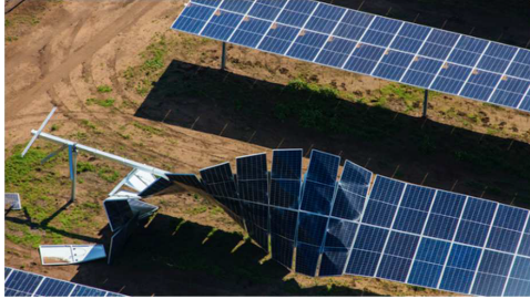
Figure 2. Single axis solar tracker facilities collapse (Source: www.pv-magazine-australia.com ).
