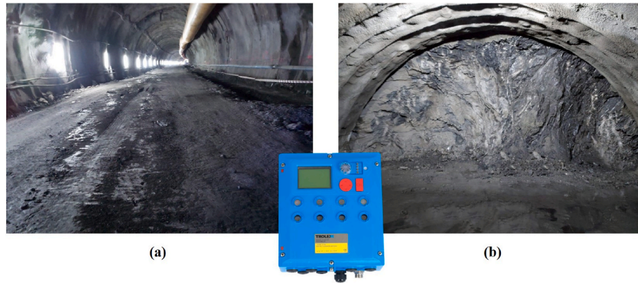
Fig. 9. Field measurements in a railway tunnel. (a) Location of flexible vent duct in the full section; (b) Top heading.
