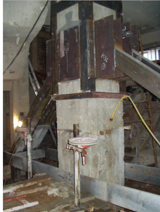
Figure 6. Cutting of the pillar using a wire saw
