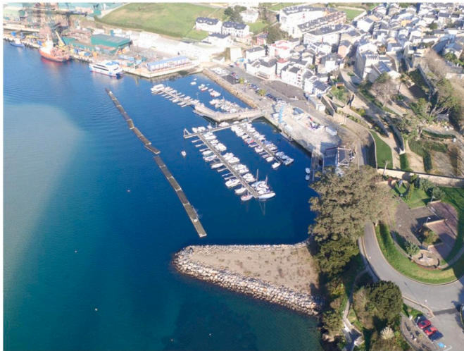
Fig. 1. Aerial photograph of the floating pontoon breakwater in Figueras marine (Asturias, Spain).
