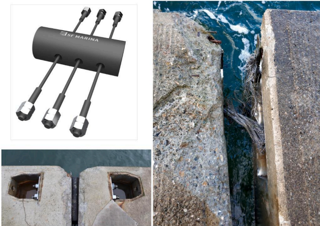
Fig. 2. Semi-rigid floating breakwater connector type (Marina) (upper left), connection installed and working properly (lower left) and broken connection after sea storms (right).
