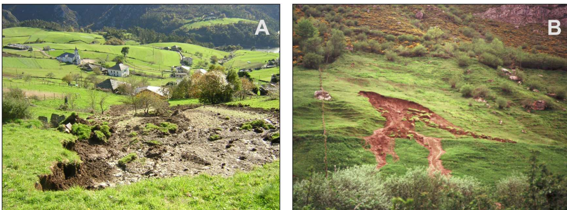
Figure 2. Some examples of rainfall-induced landslides cases in the study area. (A) Shallow landslide triggered on colluviums above slate, and (B) Shallow landslide triggered on old mass movement deposit.
