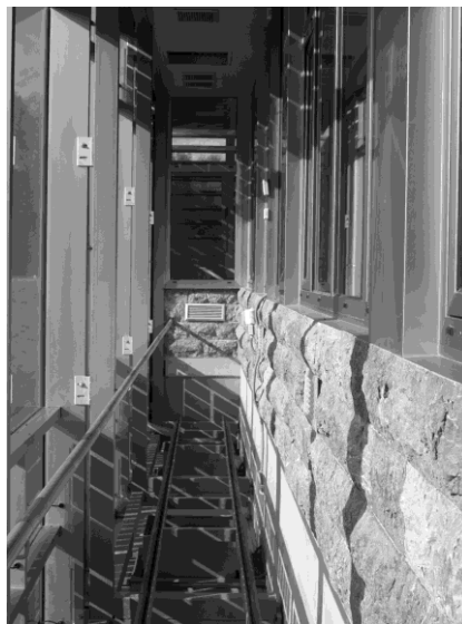
Fig. 3. Interior of the glazed gallery.
