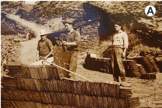
Figure 3. The beginning of the modern slate industry in Valdeorras. (A) Splitting of a slate block just in the middle of the mountain, Valley of Casaio. Photograph courtesy of Manuel Fernandez, Casaio. (B) Load of tiles directly in a truck. Photograph courtesy of Pizarras SAMACA, S.A.. This method caused many tiles to broke before arriving to destiny.
