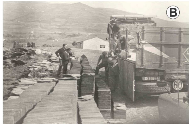
Figure 3. The beginning of the modern slate industry in Valdeorras. (A) Splitting of a slate block just in the middle of the mountain, Valley of Casaio. Photograph courtesy of Manuel Fernandez, Casaio. (B) Load of tiles directly in a truck. Photograph courtesy of Pizarras SAMACA, S.A.. This method caused many tiles to broke before arriving to destiny.
