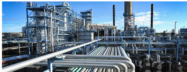
Fig. 1: Pipe racks structures
