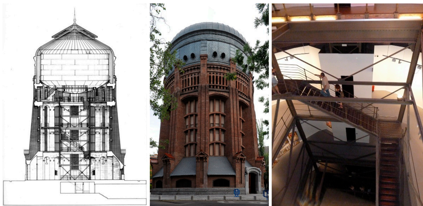
Figure 10. First water tank (1907) converted into exhibition hall (1985). Source: FMA.
