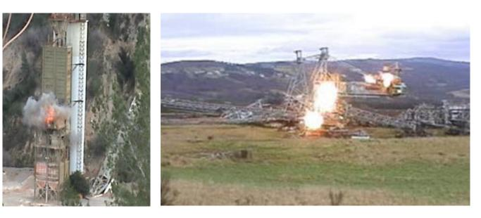
**Figure 5.** Demolition of metallic structures with shaped charges ((**left**) metallic silo; (**right**) large mining stacker).
