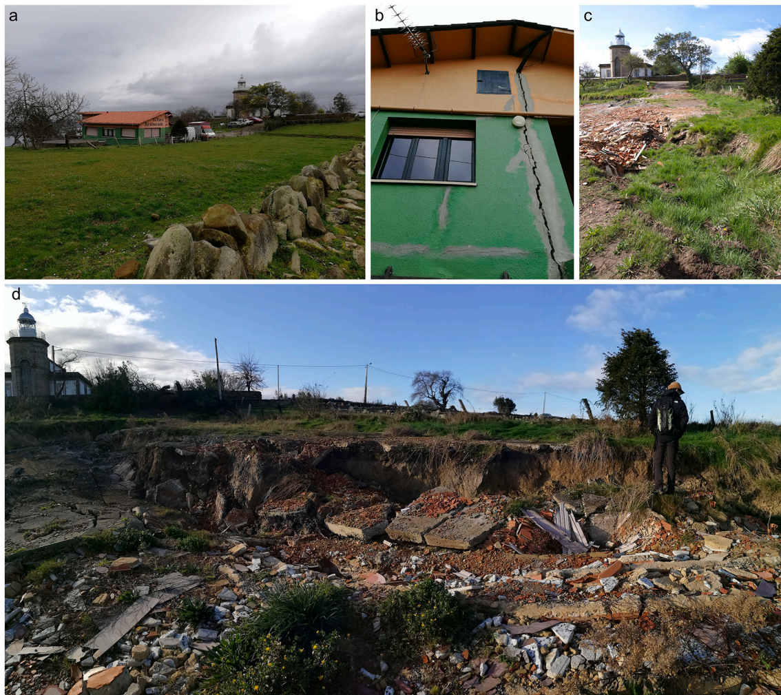
Fig. 2. a. View of the Tazones Lighthouse surroundings at the time of the restaurant eviction on February 20th 2018, after the critical enlargement of the cracks. b. Detailed view of the cracks in the restaurant building at the date of eviction. The presence of cement in the wall shows the attempt to repair old cracks that had developed before. c. d. Two views showing the evolution of surface cracks in the Tazones Lighthouse area on April 26th 2019 and January 17th 2020, respectively.
