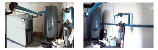
Figure 1. Piping system for the pneumatic transport.
