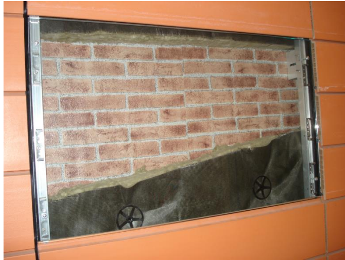
Fig. 4. Photograph of the open-joint ventilated façade structure.
