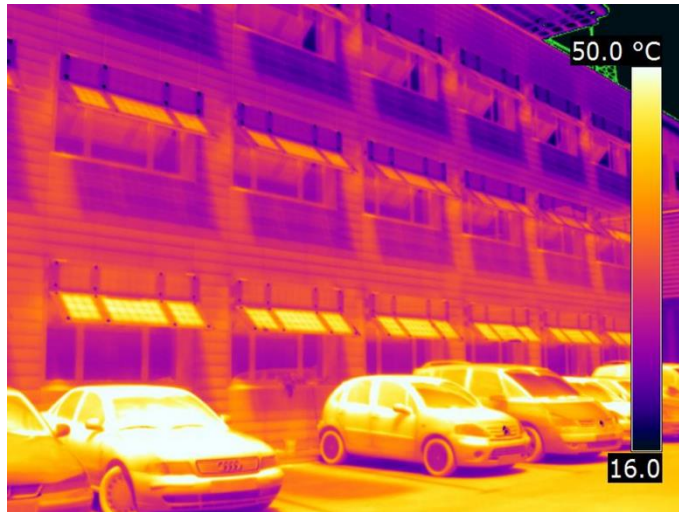
Fig. 8. Thermograph of the south façade of Madrid building, springtime, 14:00 (perpendicular solar radiation 779 \text{ W/m}^2 , exterior temperature 15.6^\circ\text{C} ).
