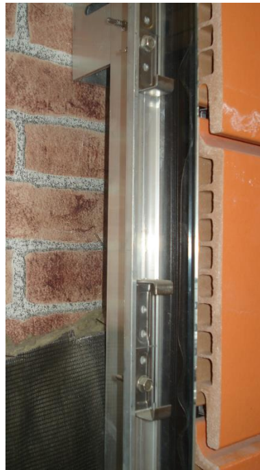
Fig. 5. Photograph of the horizontal joints detail.
