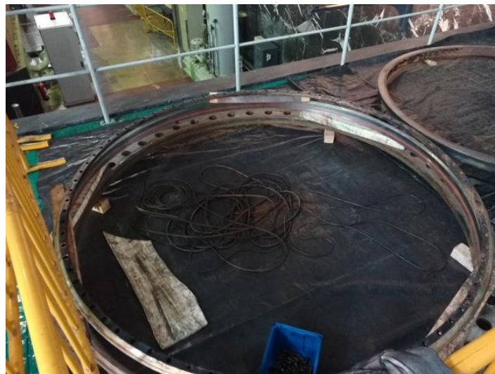
Figure 1.11: Replacement annular seal and annular seats at the Salime power house.
