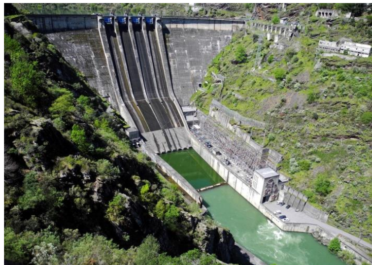
Figure 1.6: Dam, spillways, electrical substation and water discharge area of the Salime power plant
