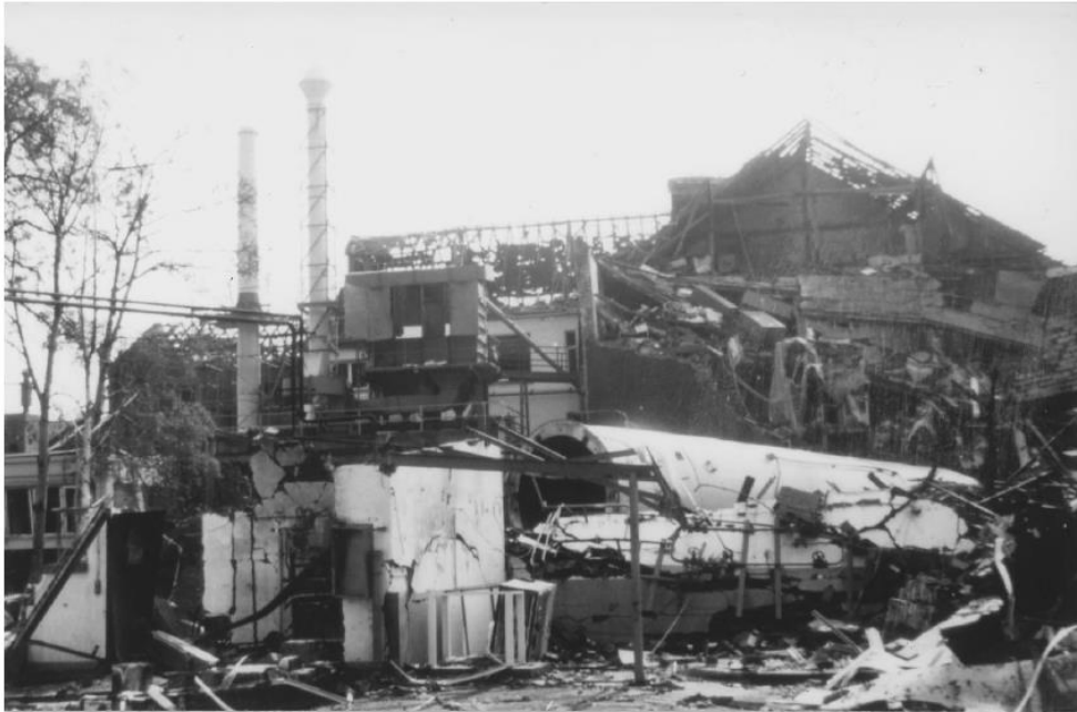
Figure 1.2. Catastrophic failure of compressed hydrogen storage tank [16].
