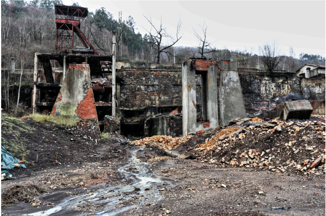
Figure 9.: Rainwater flow through the abandoned industrial installations and the brownfield, February of 2015.
