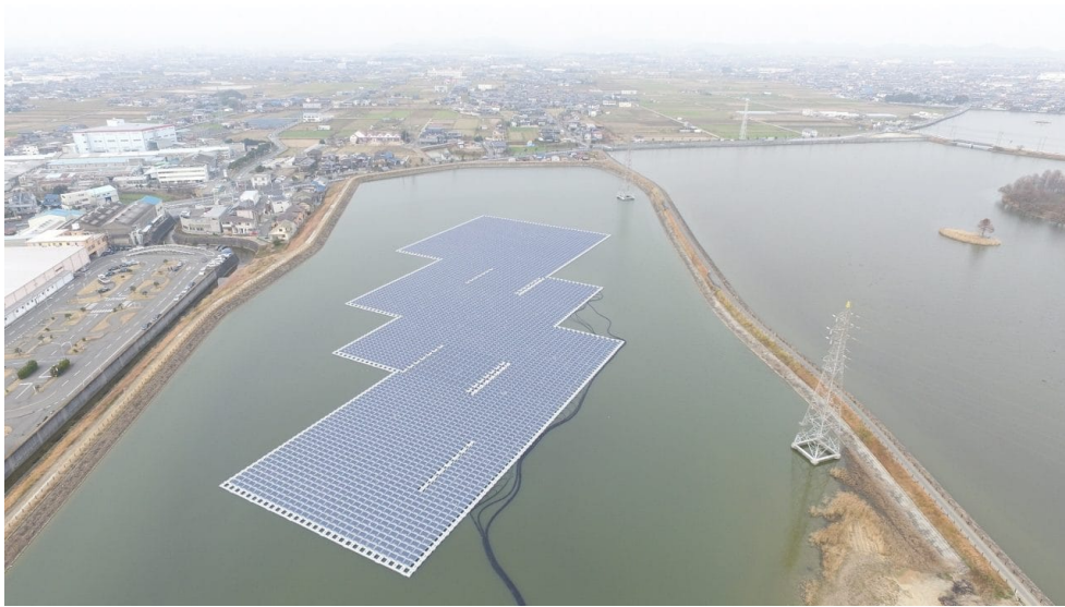
Figure 1-1: Kawarayama IKE - 1,428 kWp floating solar plant in Japan [3]
