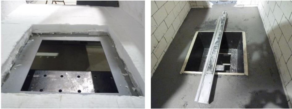
Fig. 7. Furnace floor construction.
