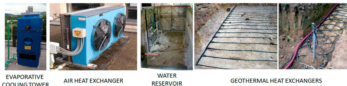
Figure 5. Heat sinks installed in the GSCL.
