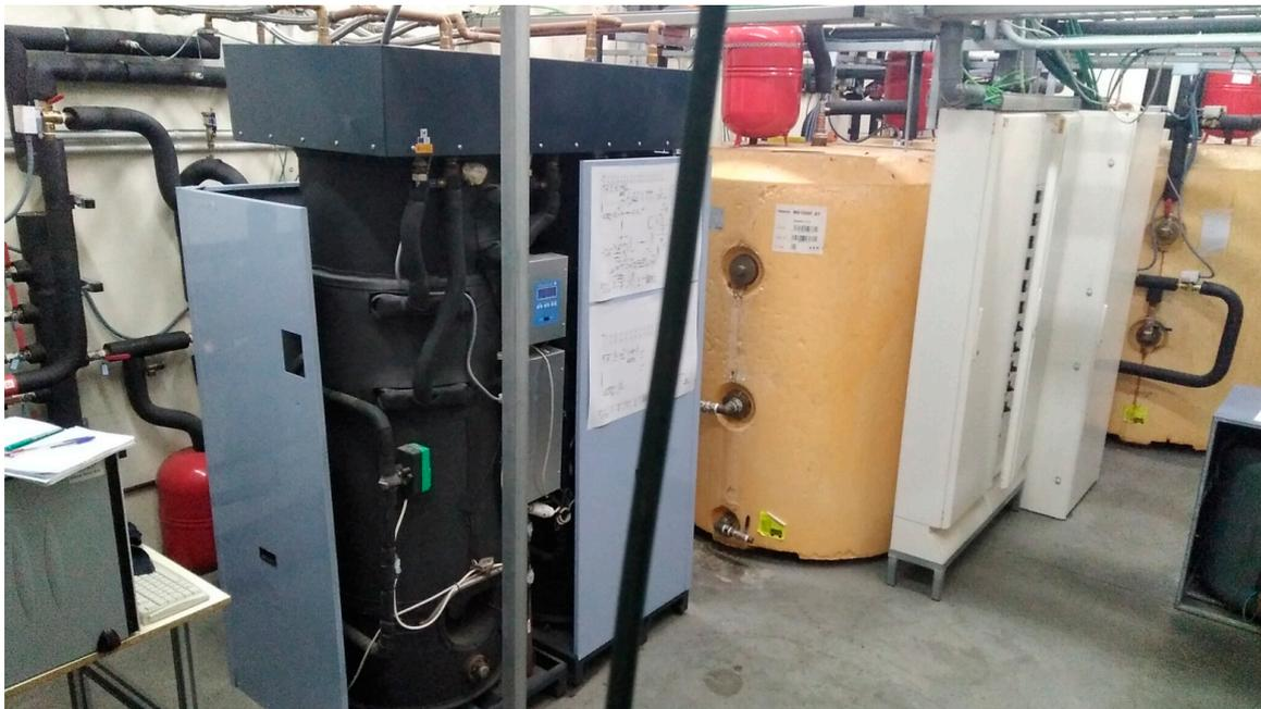
**Figure 3.** ClimateWell CW10 absorption machine installed in the GSCL.
