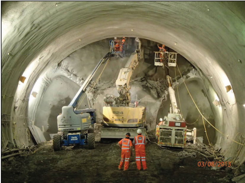
Figure 12 – WB Cavern - Installing Lattice Girders in TH of Central Enlargement
