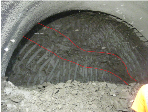
Fig. 8. Shear zone encountered between Chainages 9 and 12.
