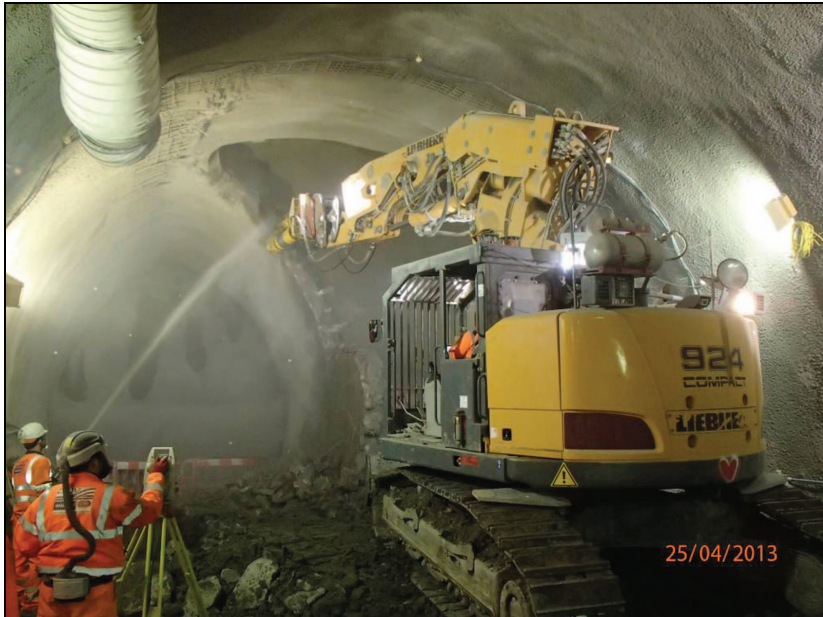
Figure 11 – EB Cavern – Removing temporary sidewall of top heading
