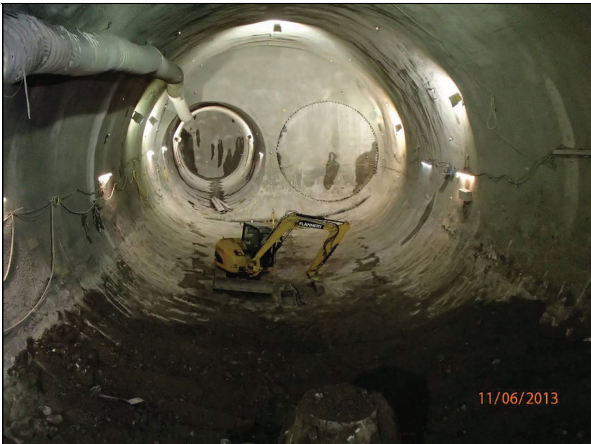
Figure 13 – Removing Backfill from Stepney Green Cavern
