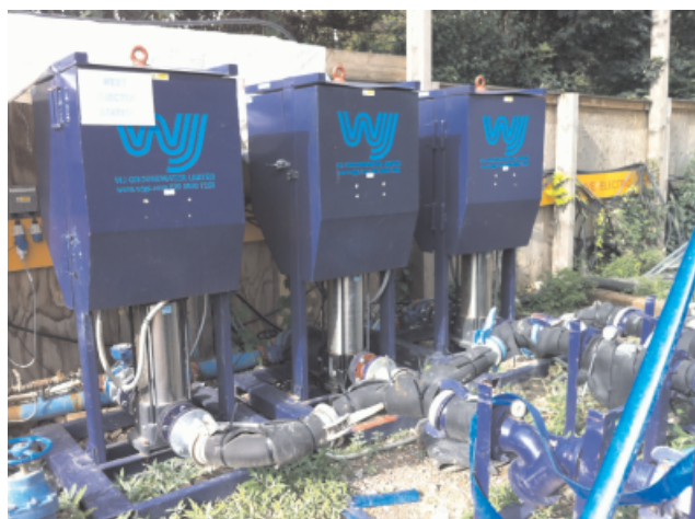
Figure 9. Multiple surface well pump arrangement
