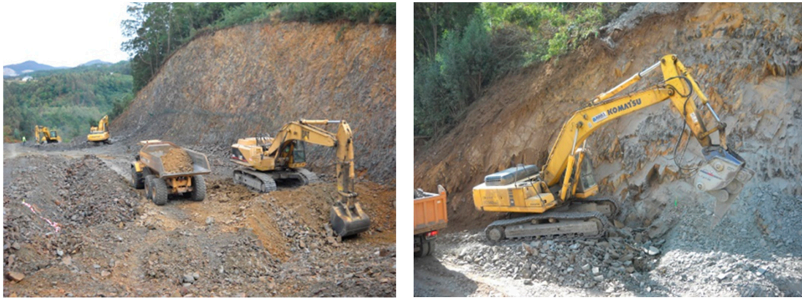
Figure 9. Machinery working in the trench.
