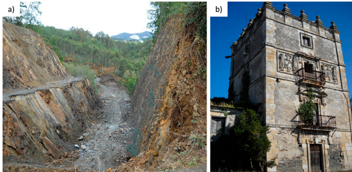
Figure 1. Case study. (a) Cut and cover tunnel under construction. (b) Historical site where the field instrumentation was placed.
