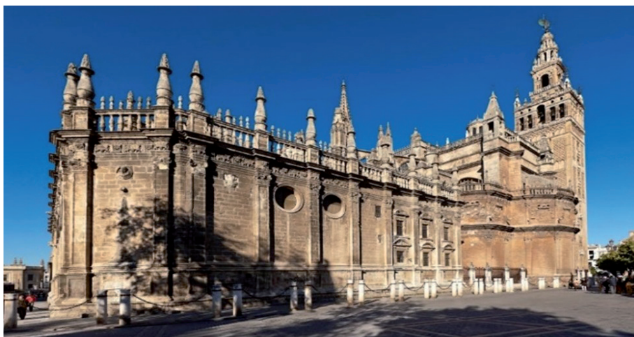
Fig. 1 General view of the Cathedral of Seville, built with sandstones of San Cristóbal (Cádiz)
