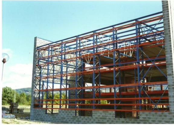
Figure 3. Structural system of self-supporting shelves, for the construction of a building
