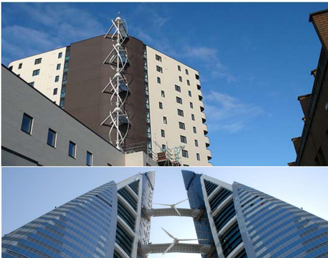
Fig 2. Sample of building-integrated turbine project [22].
