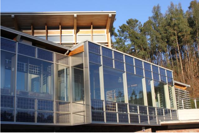
Fig. 1. Attached sunspace in demonstration-container located in the north of Spain viewed from the exterior.
