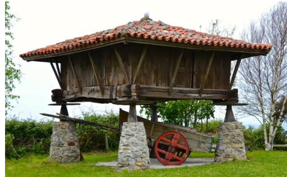
Figure 3. Horreo raised from the ground by pillars ending in flat staddle stones to prevent access by rodents. (Asturias, Spain), retaken from [2]
