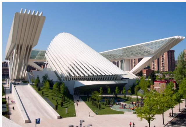
Figure 1. Congress Palace of Oviedo made of reinforcement concrete (Oviedo, Asturias, Spain), retaken from [3]
