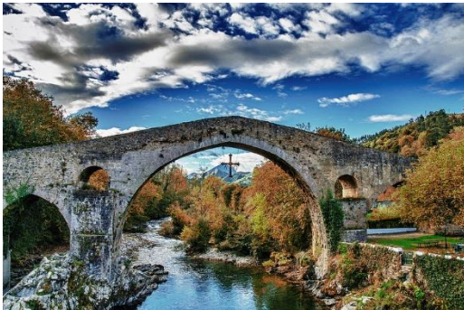
Figure 2. Roman bridge built with stone with an arch as its basic structure. (see e.g. Cangas de Onís, Asturias, Spain) retaken from [1]
