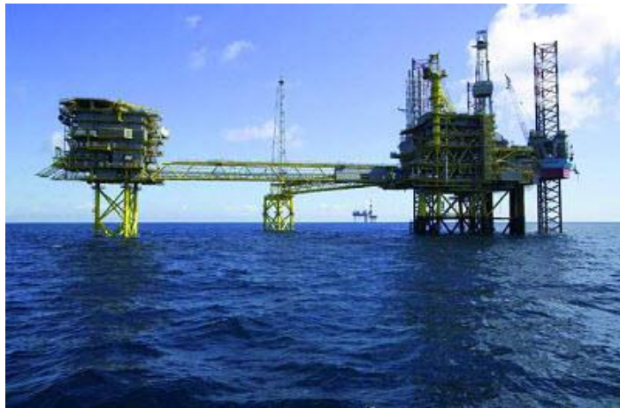
Figure 2.13 Oil installation in a harsh marine environment
