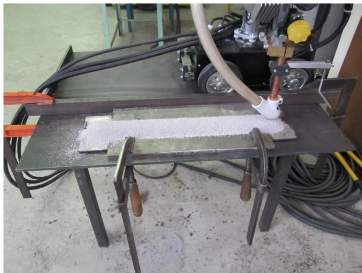
Fig.5.6. Welding process of test joint
