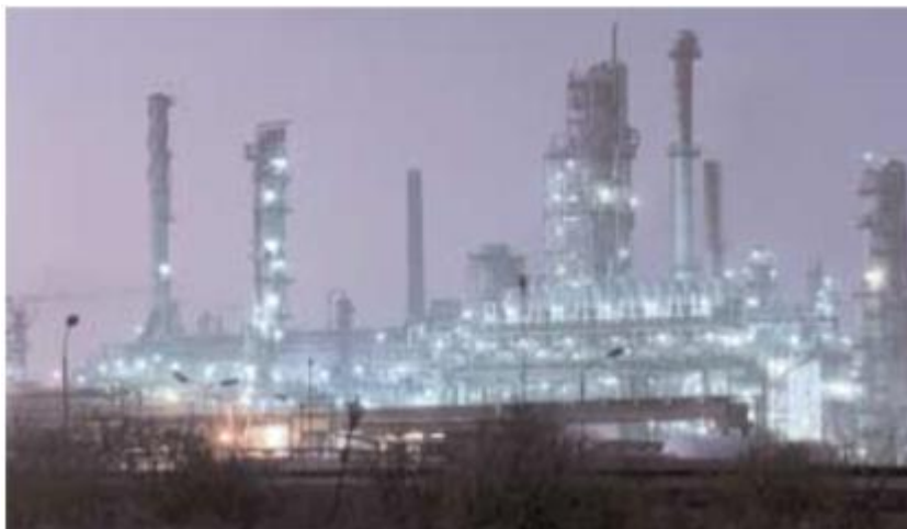
Figure 2.1 Chemical Processing Plant of duplex stainless steel
