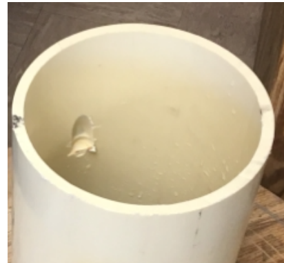
Fig. 7. PVC pipe with internal damage.
