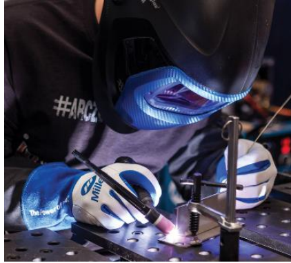
Figure 26. Welder executing GTAW welding.
