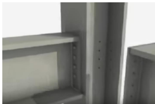
Fig. 2.4. Beam to column connection with the flange and web of the column.
