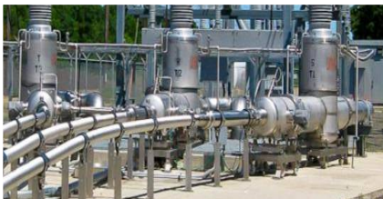
Figura 3-2: Cable superconductor
