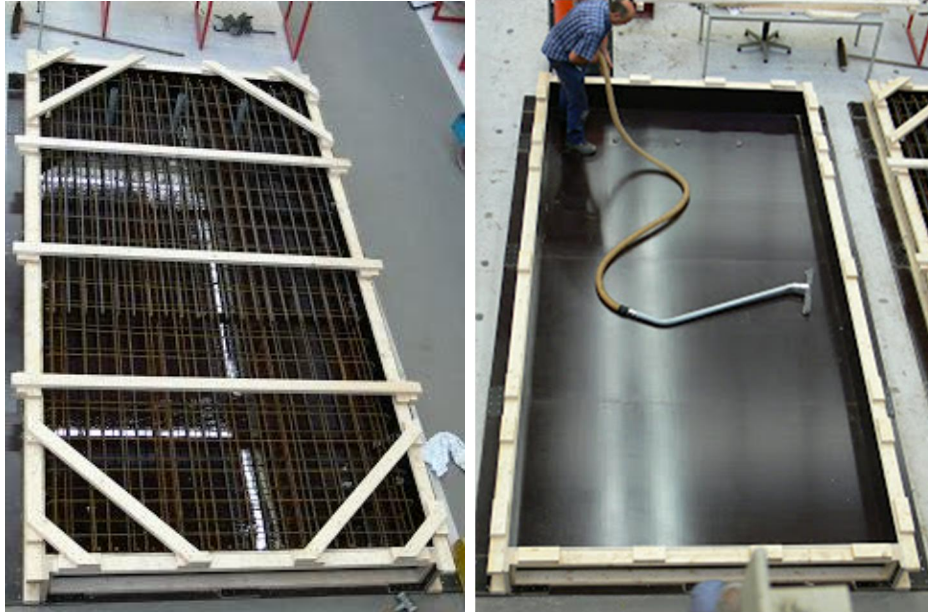
Figure 4: Reinforcing bars placed at the formwork (1) and concrete vibrator machine (2)
