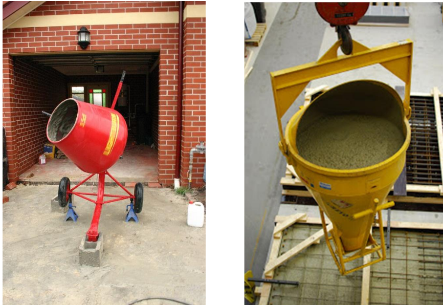
Figure 3: Concrete mixer (1) and mix falling down by gravity into the formwork (2)
