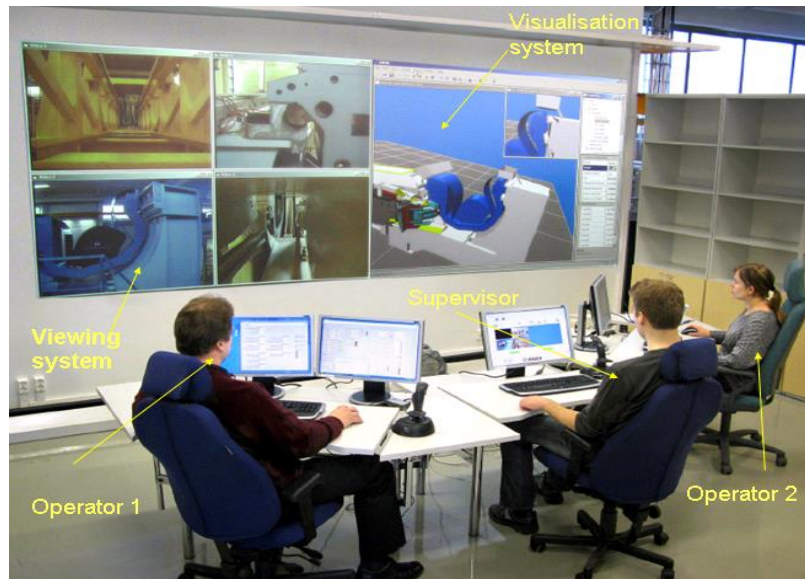
Fig. 186. DTP2 control room.
