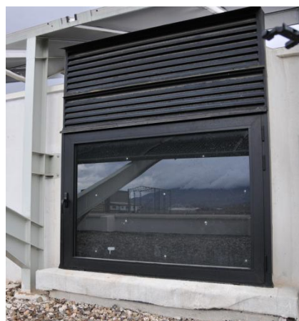
Fig. 1. CIEMAT research building at Almería's Solar Platform. Solar chimney detail.
