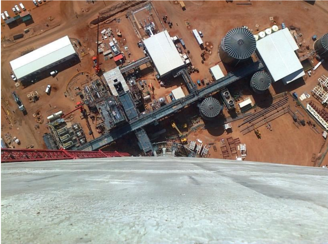
Figure 3.13. Top view of the power block. Image: IMASA.
