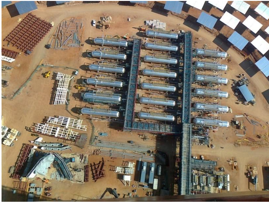
Fig. 3.7 Steam Accumulator Tanks. Image: IMASA.
