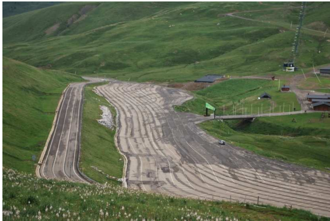
Figure 4.- Creep phenomena in the parking-lot area.
