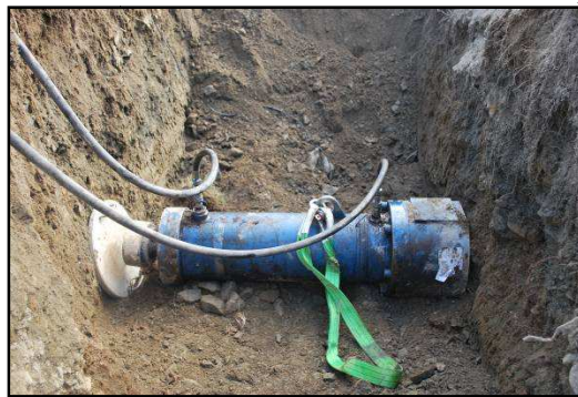
Figure 6- Hydraulic cylinder placed in a trench
