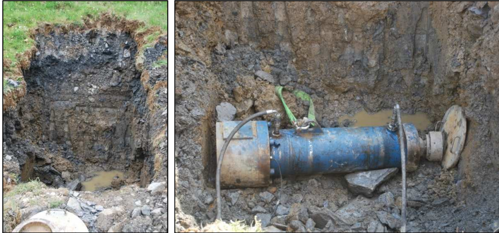
Figure 13.- State of one of the excavated trenches for the on-site tests
