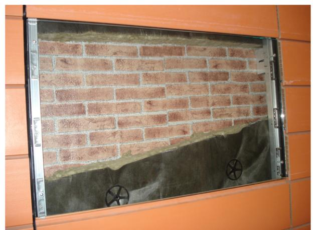
Fig. 4. Photograph of the open-joint ventilated façade structure.
