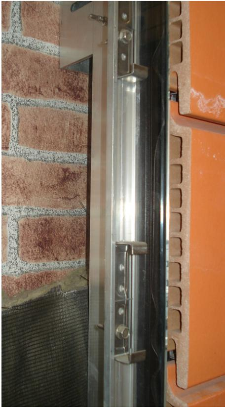
Fig. 5. Photograph of the horizontal joints detail.
