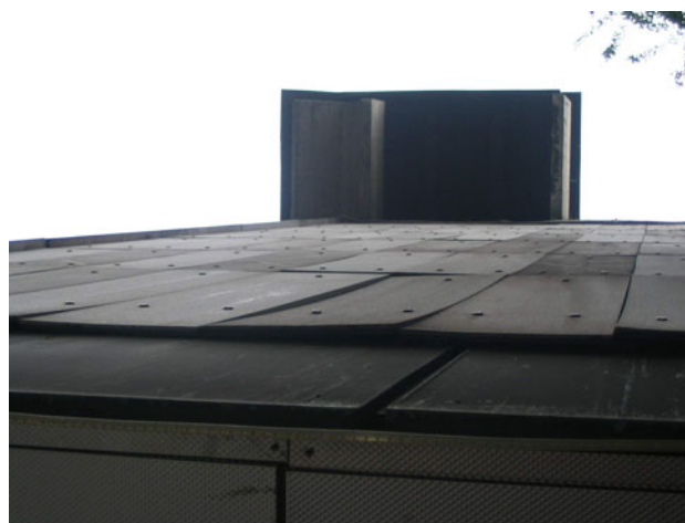
Fig. 1 Cezlak granodiotite showing bowing
