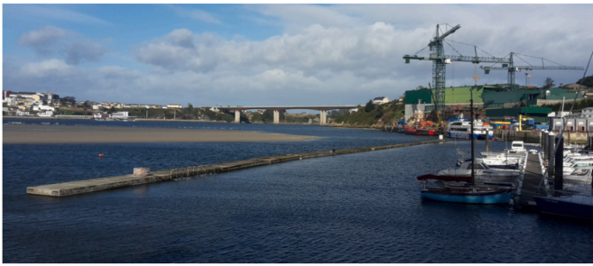
Fig. 1. Pontoon-type floating breakwater in the Port of Figueras (Asturias, Spain).
