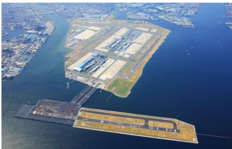
Figura 37. Haneda International Airport, Tokyo [130].
