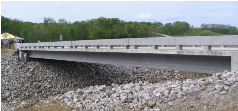
Figura 31. Mars Hill Bridge, Wapello County, IA [11].
