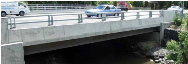
Figura 35. The Shepherds Creek bridge, Australia [129].
