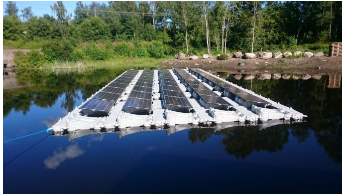
(a) Pure float floating system [1]
