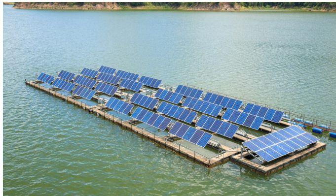
(b) Pontoon type floating system [6]
