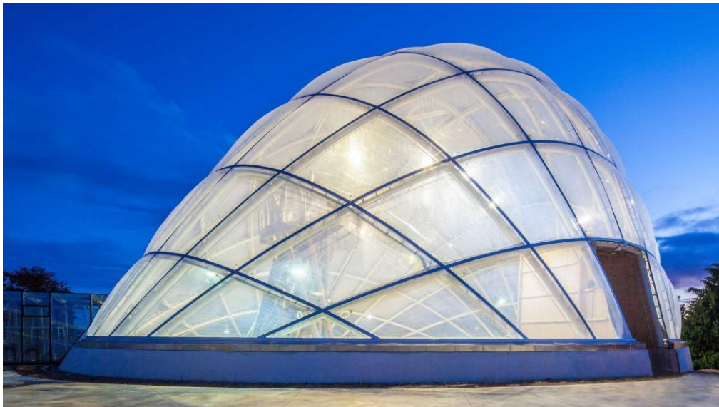
Figure 3.28. EFTE in building structures
