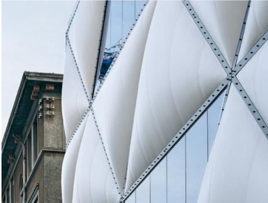
Figure 3.29. PETG in building structures
