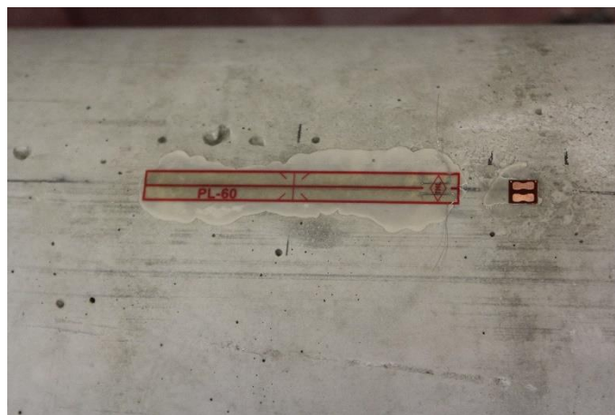
Figure 3.37-Final placement of strain gauges.
