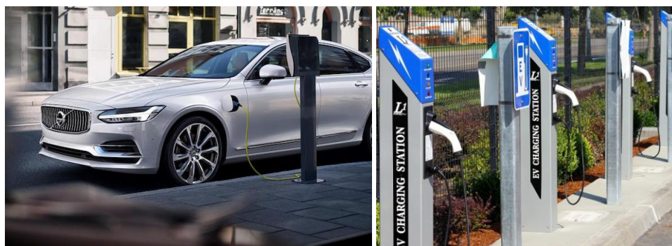
Figure 32 LHS A charge point with EV connected. RHS A collection of points comprising a charge station [58] [59].
