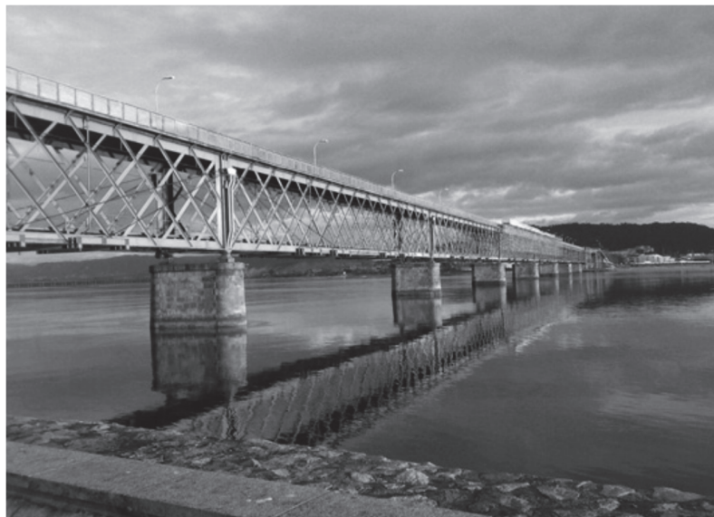
Figure 5: Riveted metallic Eiffel bridge in Viana do Castelo (Portugal).
