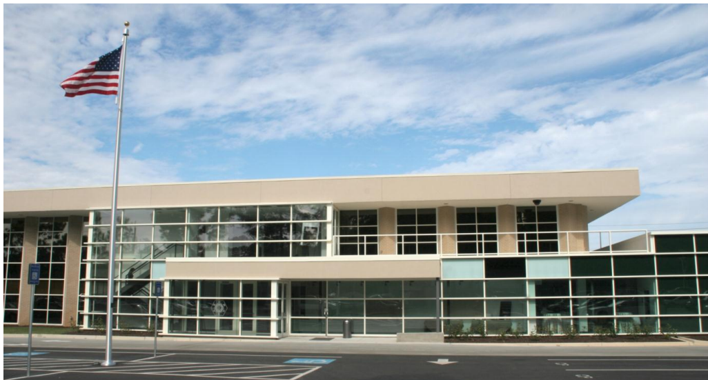
Figure 10. ASHRAE HQ Building at Atlanta, GA. (P. Konečný, L.E. Southard, Spitler, C., 2014)
