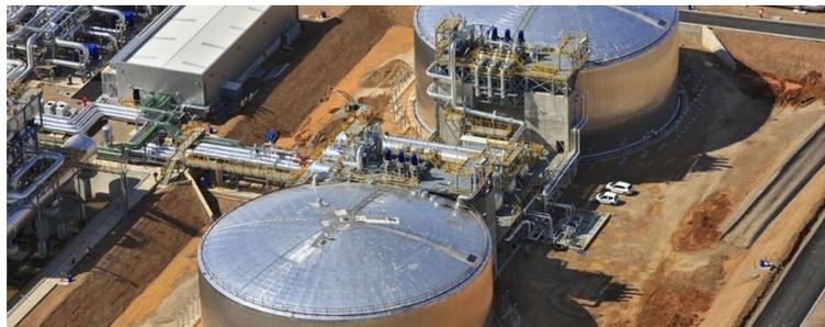
**Figure 1.** Molten salt tanks for storing thermal energy in the solar plant “La Africana” Granada.
