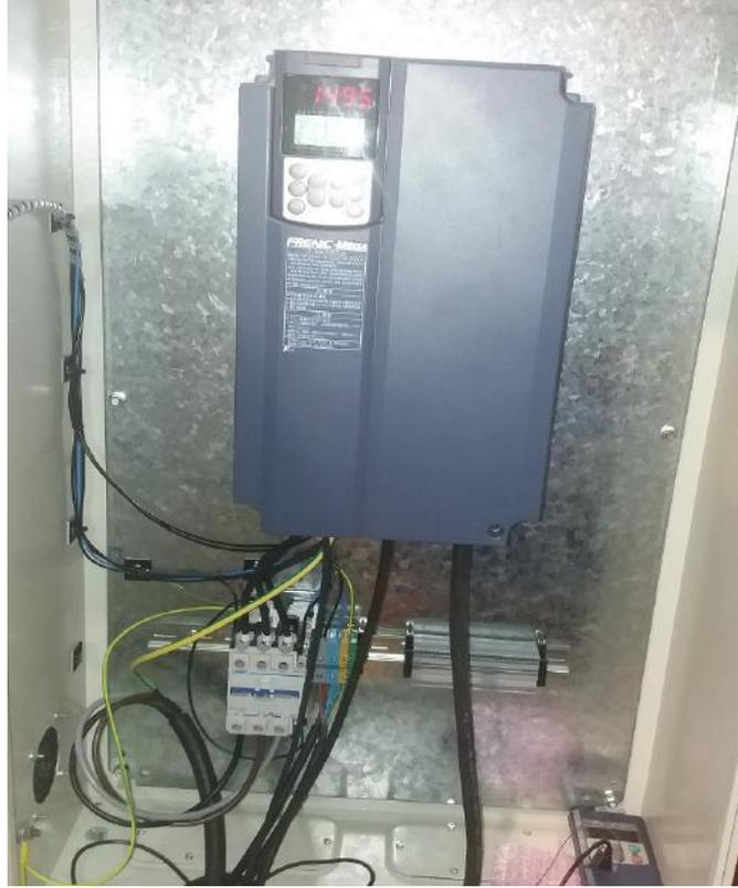
Figure 5-5: Commercial electric drive for prime mover
